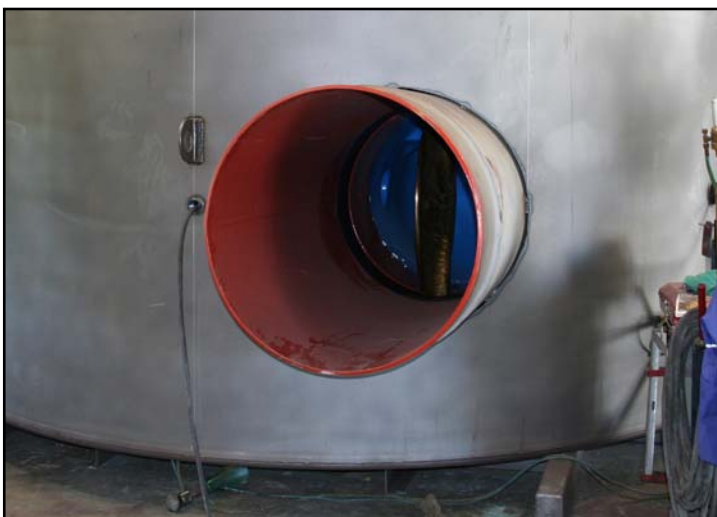
This picture shows the piping coming through the capsule sidewall and tack welded into place prior to the inside and outside seal welding operation. The transmission pipe at the capsule shell weld joint has a 2" thick steel sleeve welded over it where it passes through the capsule wall; this sleeve pipe lining is attached prior to fusion bonding the pipe serves as a heat sink to keep the capsule seal weld heat from burning the fusion-bonded epoxy.
