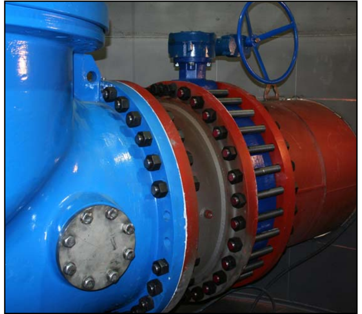
This picture shows the 36" valve assembled into the transmission piping with the inlet-side isolation, wafer butterfly valve.
