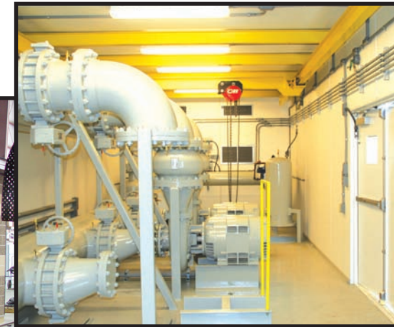
Mechanical and electrical equipment mounted to the steel base and to the sidewalls
