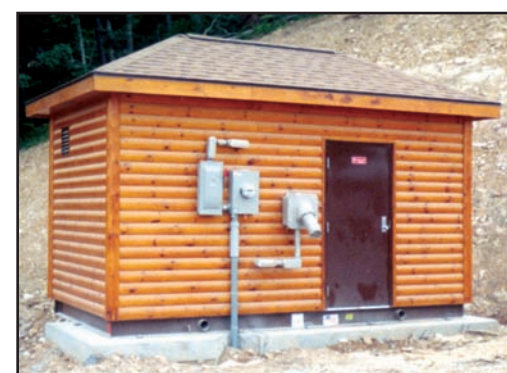
Wood Siding with a Shingled, Hip Roof.
