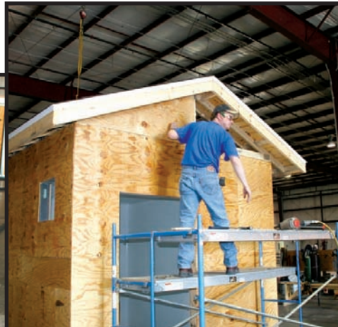
Building in final assembly
