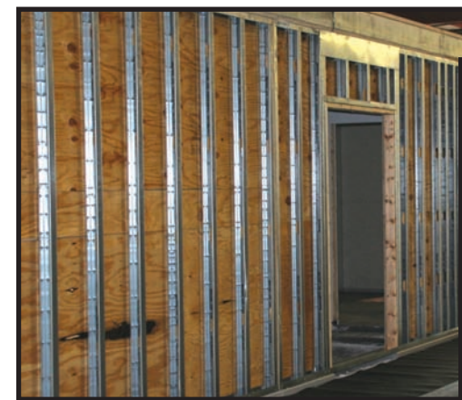
Jig built, ASTM steel framing for walls & ceiling with interior plywood sheathing
