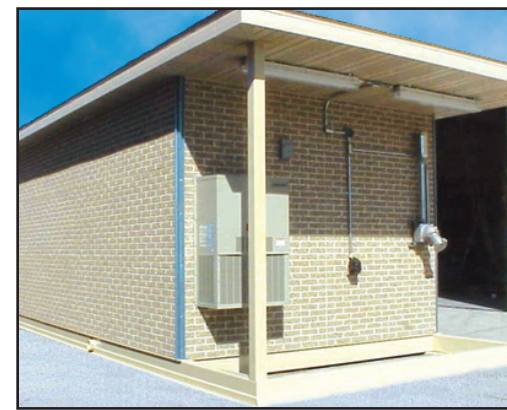
Factory Applied Staggered Brick Panels with a Hip Roof w/overhang for generator hookup.
