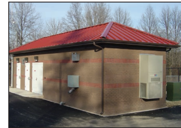
Field Installed Brick with a Standing Seam Metal Roof.
