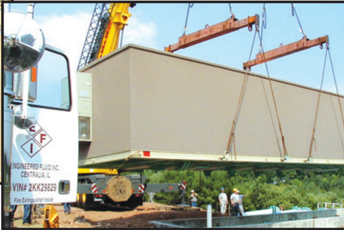
Field setting of EFI delivered building over a foundation
