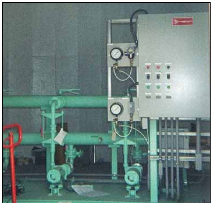
Here shown is a view into the elevated tank base showing the skid, tri-plex booster station and pump controls.
