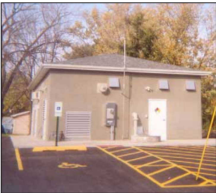
Here shown is the the finished installation with the roof complete, the fascia, soffits, gutters, downspouts, and seam strips attached. The three doors, rear to front, are the pre-treatment chlorine feed room, the office and control room, and the stand-by generator room to the front.
