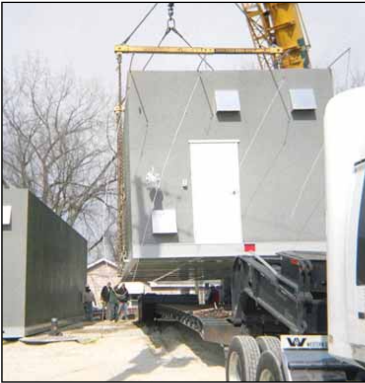
Here shown is the eastern half of the treatment facility being lifted for placement on the foundation next to the western half.
