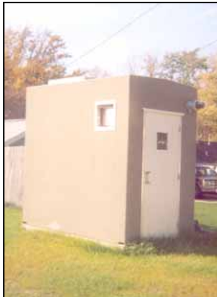
Here shown is one of the new well-houses fabricated complete and installed over the well head following demolition of the old well house.
